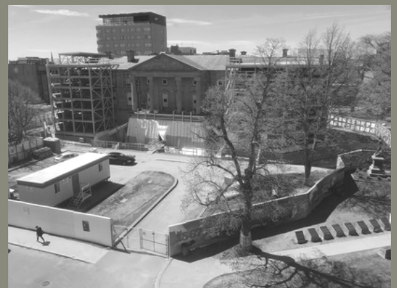
Province House under construction, the view from the attic.
